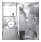
Other analog manometers also known as Magnehelic® Gauges have been around for decades. They're very durable, they hold their calibration well, and provide a very direct static pressure reading through a needle gauge. The down side is they need to be perfectly level to get accurate readings – often difficult to do
